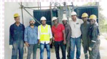
Successfully Installation, Testing and Pre-commissioning work completed - Indorama Ventures PET Nigeria Ltd at Port Harcourt (Nigeria)
