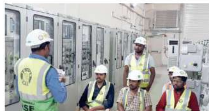
Jeriyan Jenaihat-1 Substation, Qatar
