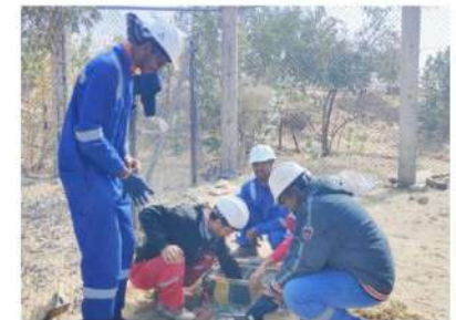
Our Engineers Testing the Earth Pits at Cairn India Ltd, Barmer
