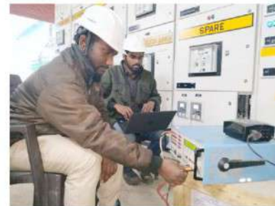
Our Engineer Mr. Saravana Kumar & Mr. Karunagarar testing the relays at 4x210 MW NTPC, Dabri
