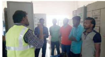
SIEMENS - Ranchi (Eastern Region)
