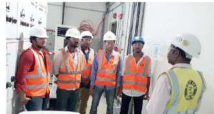
New Assiri Substation, Qatar
